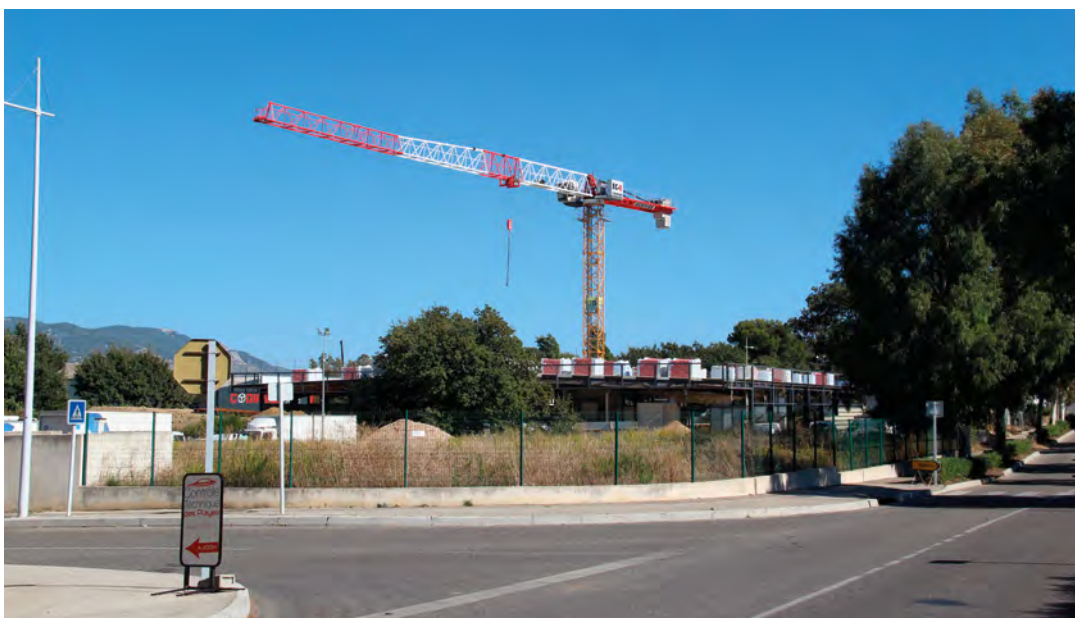
Construction Molly Bracken
